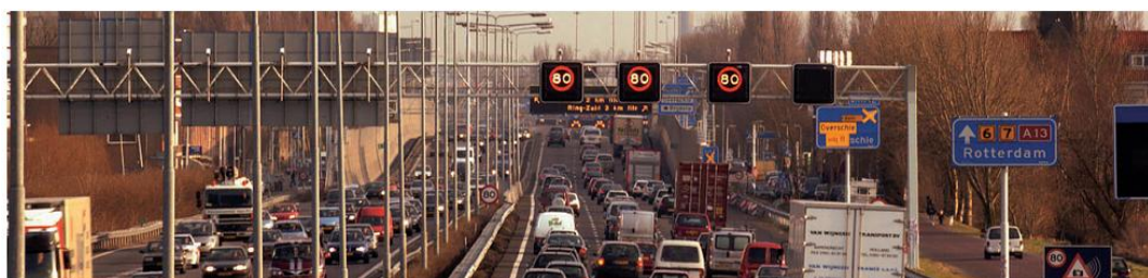
Figure B.1: 3 road signs consist the enforcement part of the Dynamax system.
